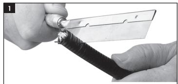
Cut the cable square. If necessary, bend the cable slightly at about 5" (127 mm) for more gripping leverage. **Note:** Do not exceed the minimum bend radius of the cable.
